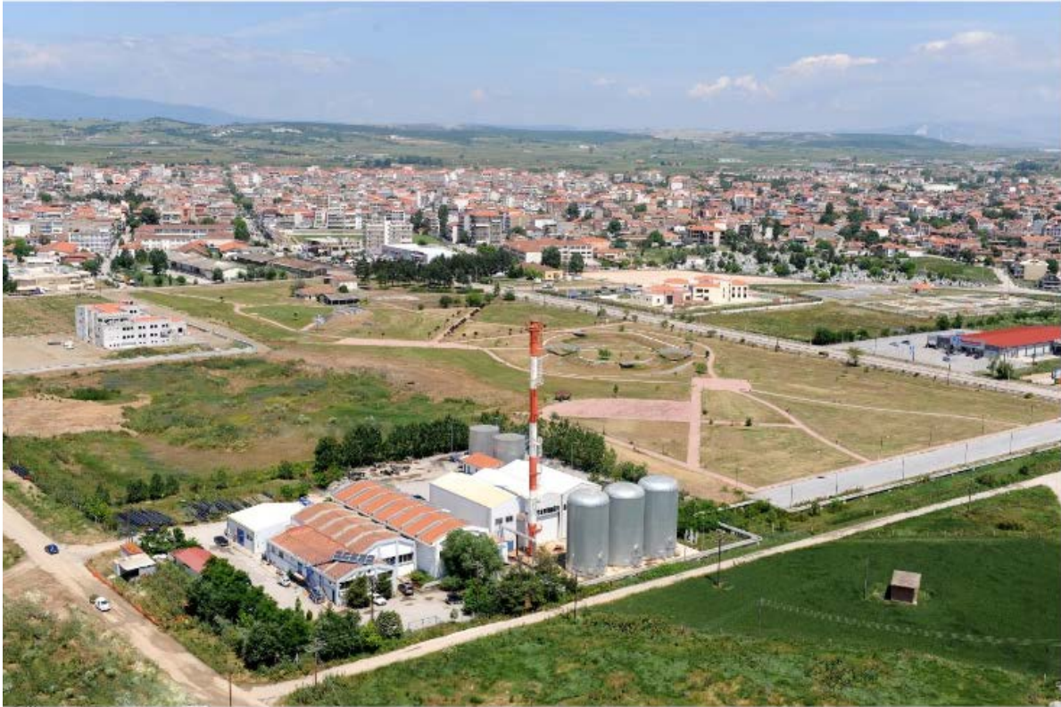
Image 1.2: Central pump house of the Public Enterprise for District Heating in Ptolemaida (DETIP) at the southern entrance of Ptolemaida 2
