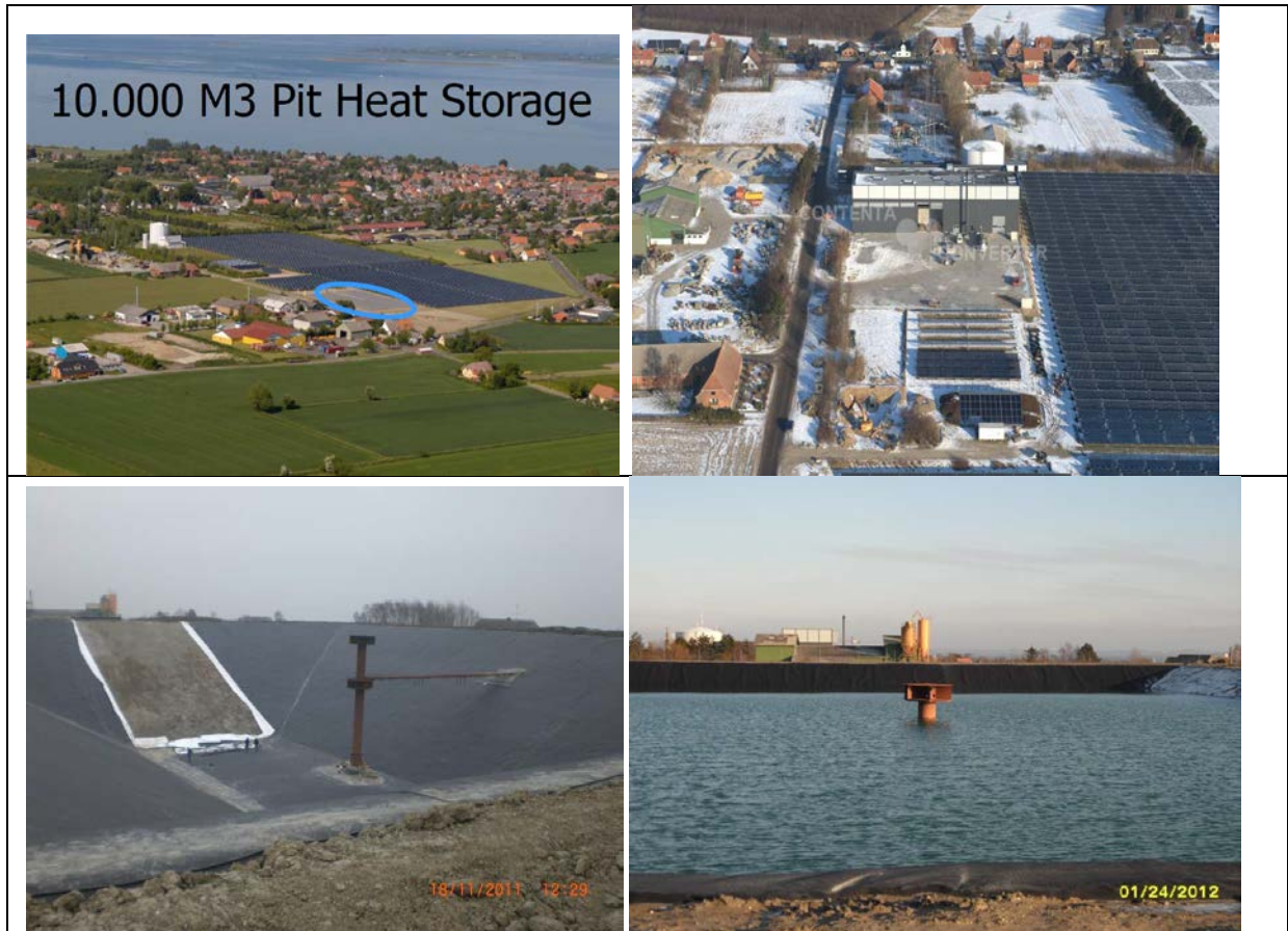
Image 1.4: Solar farm and seasonal heat storage in the city of Marstal, Denmark 19
