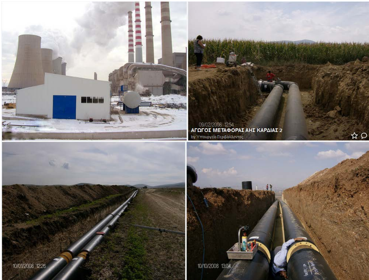
Image 1.1: District heating in Ptolemaida - Connection with the steam-electric power station at Kardias 1
